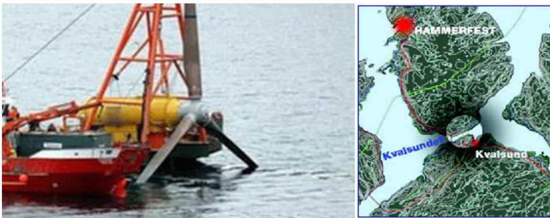
Deployment of the first grid connected marine turbine in Kvalsundet (Norway)
